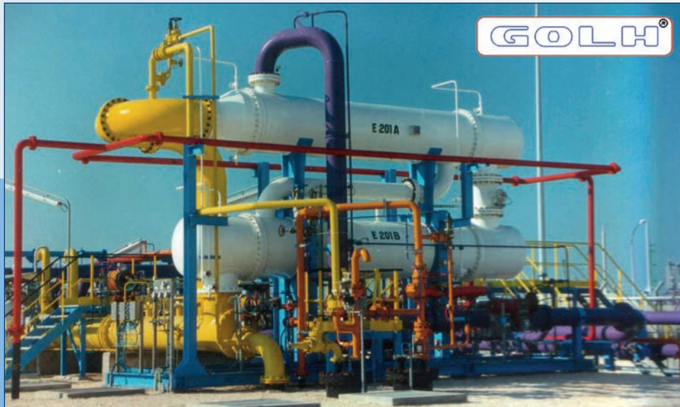
G.O.L.H. ® Gas On Line Heating system suitable for cryogenic LPG heating by sea water.
