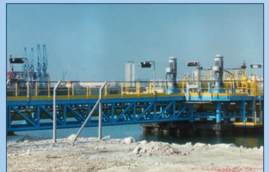
Sea water intake
